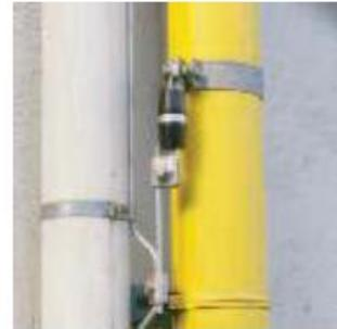
Spark gaps 480 and 481 are installed with attaching straps or connectors between the system parts to be bridged. When installing, cable lengths should be kept as short as possible, as long cables increase the risk of insulation being subjected to unnecessary demands through inductive voltages.
